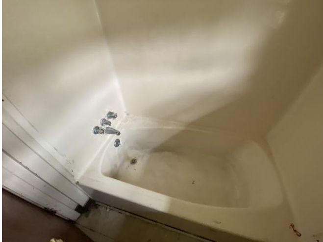
Bathroom (being held for renovations) (view one of two)
