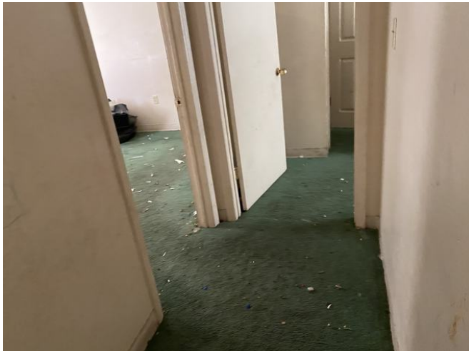
In-unit hallway (being held for renovations)
