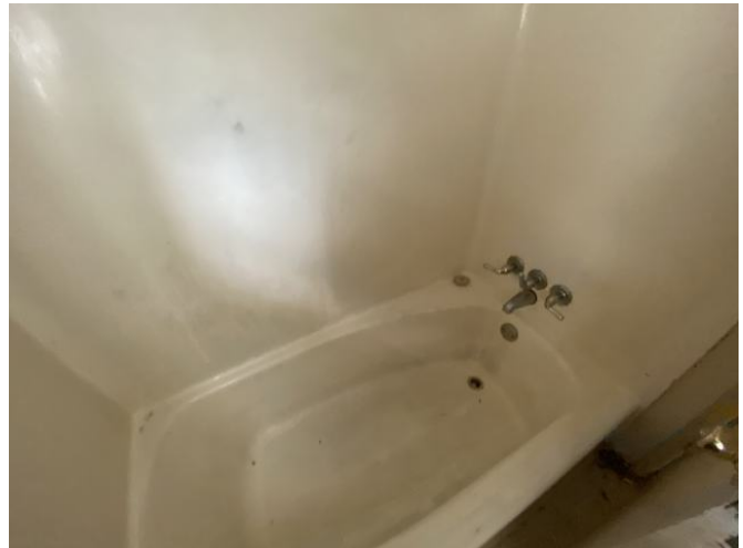
Bathroom (being held for renovations)
