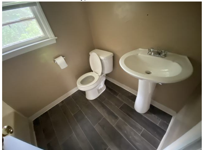
Typical bathroom (view one of two)
