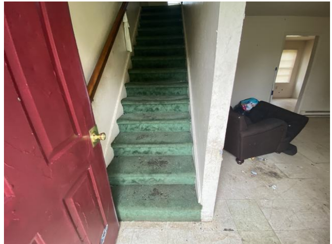
In-unit staircase (being held for renovations)
