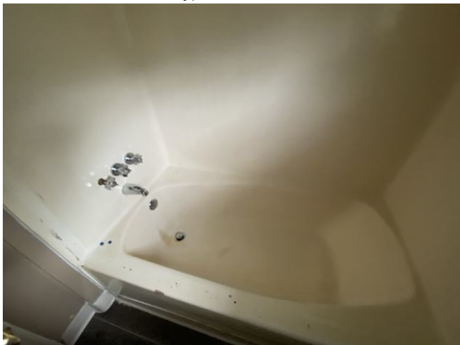
Typical bathroom (view two of two)
