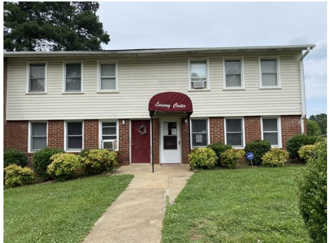
Leasing office exterior
