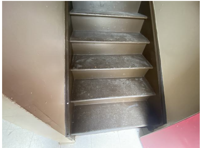
Typical in-unit staircase
