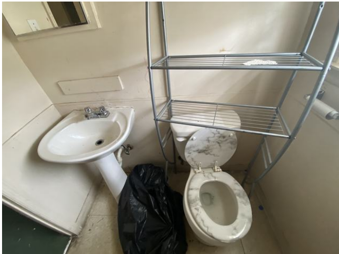
Bathroom (being held for renovations)
