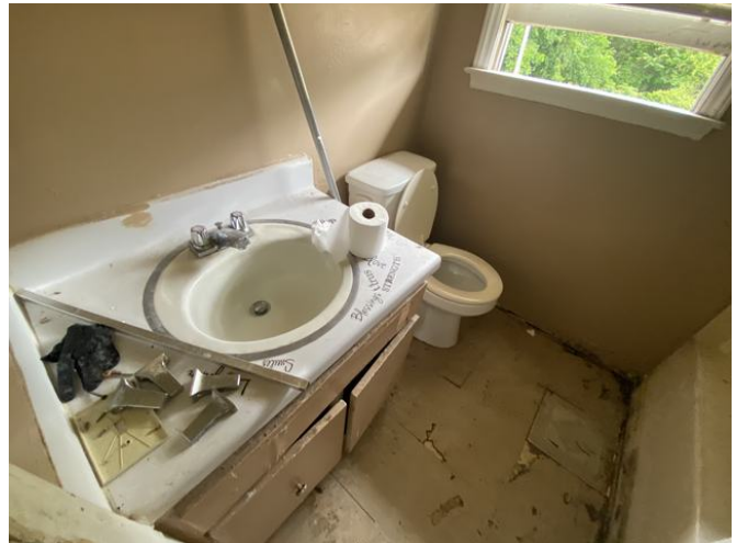
Bathroom (being held for renovations)
