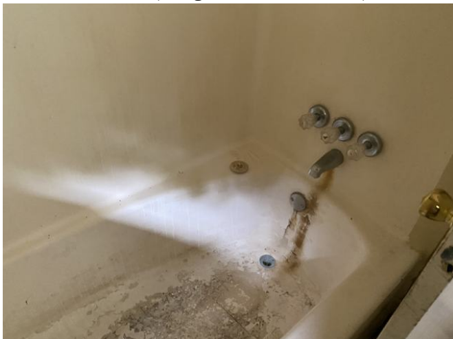
Bathroom (being held for renovations)
